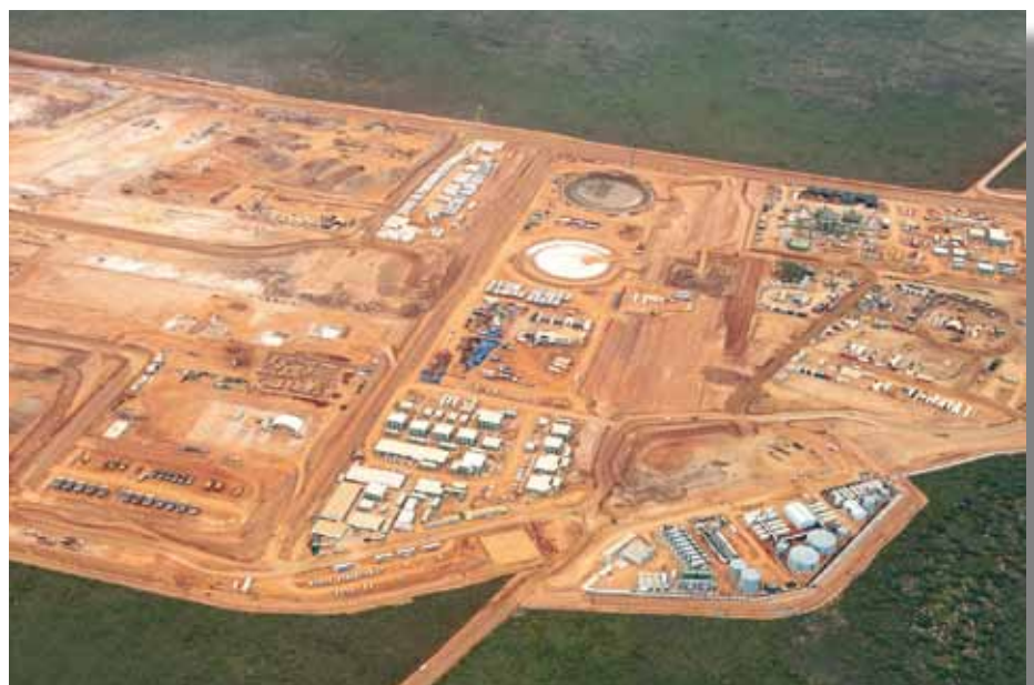
Chevron Gorgon LNG plant under construction on Barrow Island.
