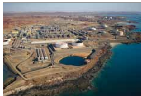
Woodside Burrup Peninsula plant.
