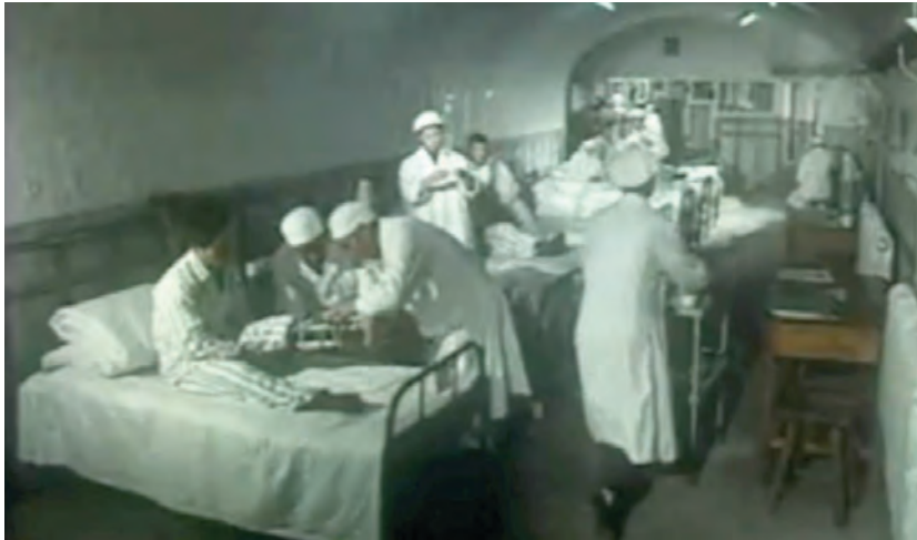
Active hospital in underground city
