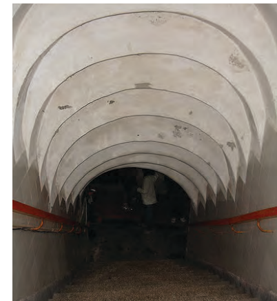
Staircase descending 8-18 meters.
