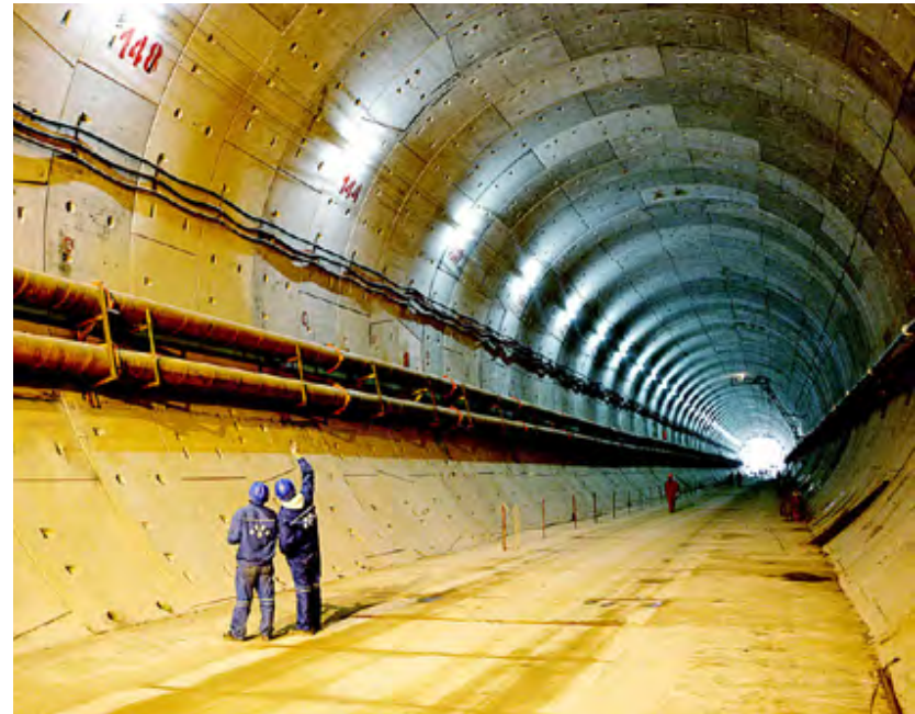
Shanghai Yangtze River Tunnel
