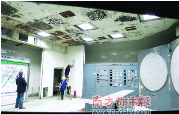
Control Room under repair
