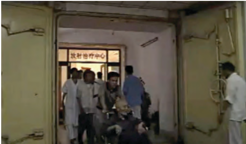
Heavy blast/anti-radiation doors on underground hospital
