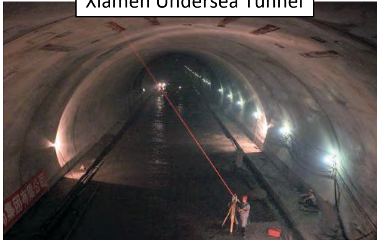
Xiamen Undersea Tunnel
